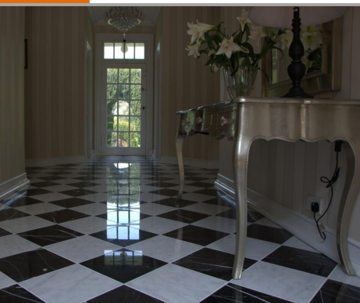
Black and white marble tiles bonded to a DITRA mat.
